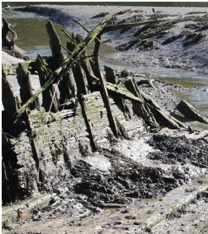
FIGURE 9: THE STARBOARD SIDE IN 2016, SHOWING THE CHANGES SINCE 2007: MUCH OF THE PLANKING HAS BEEN LOST AND THE DECKING THAT PREVIOUSLY RESTED ON THE KNEE HAS ALSO GONE.
