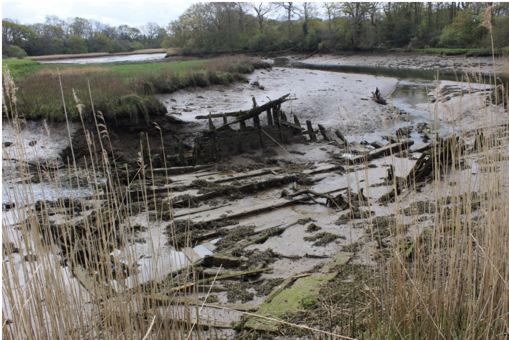
FIGURE 2: HULK OF THE BARGE WESSEX SITTING IN A TRIBUTARY OFF THE MAIN HAMBLE RIVER.
