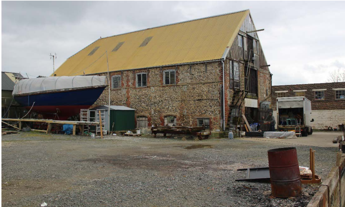
FIGURE 6: EXTERNAL IMAGE OF LITTLEHAMPTONS SHIPBUILDERS.
